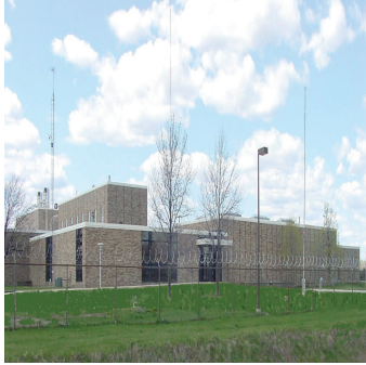
City of Oregon Water Treatment Plant
