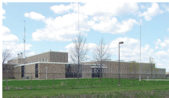
City of Oregon Water Treatment Plant
