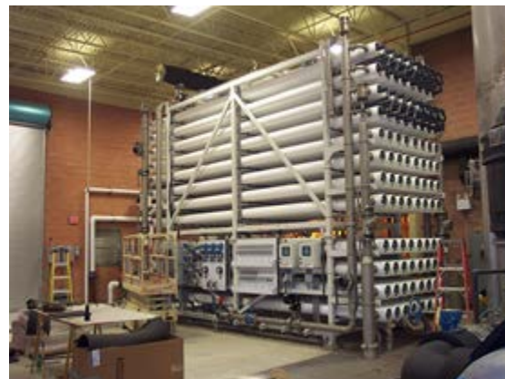
City of Bowling Green Water Treatment Plant
