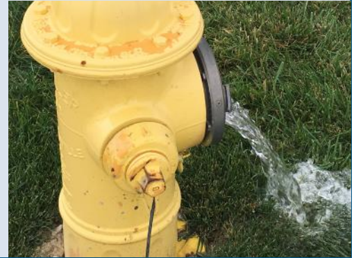
Pictured above: Water from a hydrant at the beginning of the flush. Pictured below: The same hydrant minutes later. The process involves letting the water run but also checking valves, bolts and all parts that allow this important first-responder tool to continue working.
