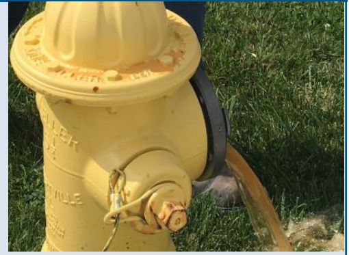
Pictured above: Water from a hydrant at the beginning of the flush. Pictured below: The same hydrant minutes later. The process involves letting the water run but also checking valves, bolts and all parts that allow this important first-responder tool to continue working.
