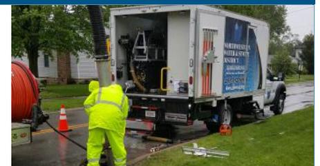
Above: From the Technology story, The District camera truck and vac truck work together to collect system data.
