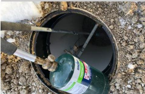
Above Photo: Photograph of a newly installed meter pit in Rossford as part of the lead service line replacement project. Crews are seen above heating the pit to prevent it from freezing in the cold weather.
