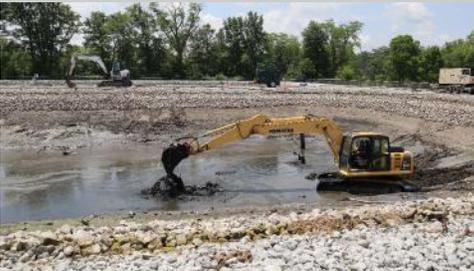
Above: The District is investing \$200,000 on a unique project at our Tontogany Wastewater Treatment Plant. This picture shows maintenance work to remove sludge from the bottom of our lagoons. This three week project involved draining two lagoons then "dewatering" the sludge to be disposed of at a landfill.
