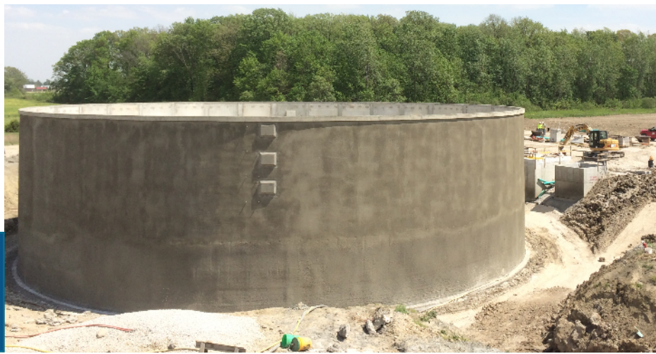
Photo of the EQ Basin in Northwood this June. More on how it improves water quality in Northwest Ohio on page 2.
